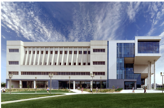
Glass Hall Renovation and Addition completed in October 2017. Photo Courtesy of Gayle Babcock.
