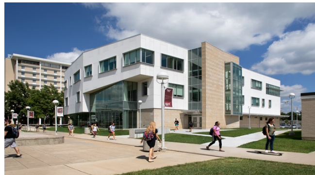
Magers Health & Wellness Center completed in April 2018.
