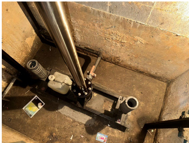
The Elevator No. 16 Pit, Jack Unit, & Spring Buffers
