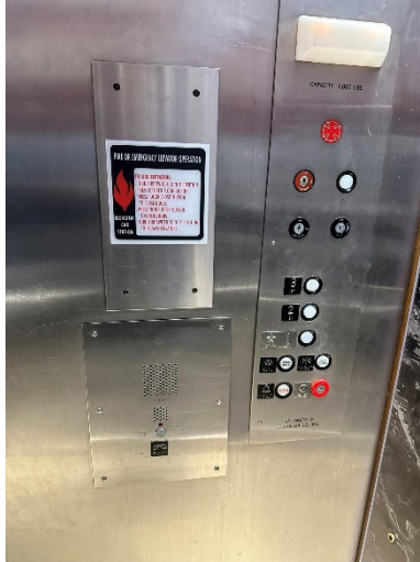
Car Control Station for Elevator No. 16
