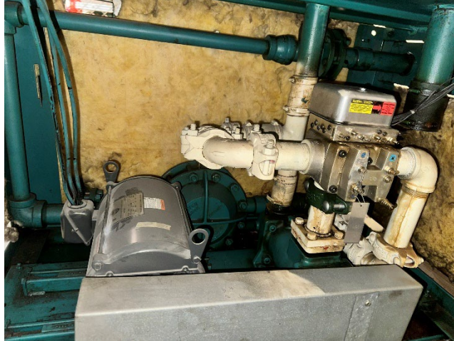
View of the Pump, Motor, and Maxton Control Valve
