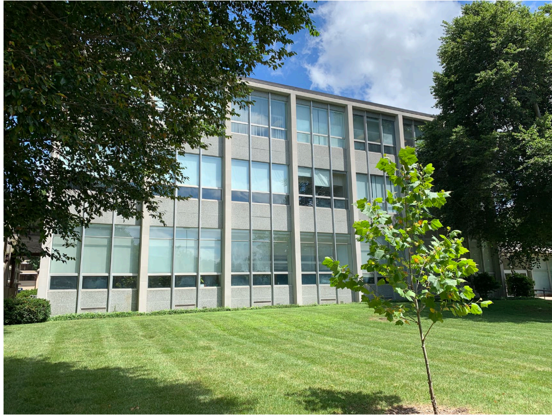
South elevation of Cheek Hall (above and above right).
