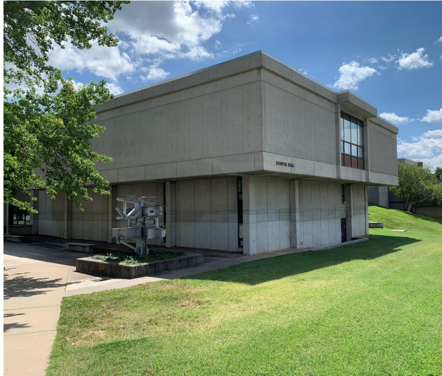
Main elevation of Kemper Hall (above).
